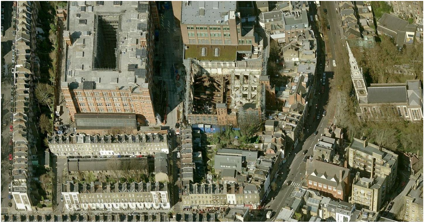
Aerial view of the site
